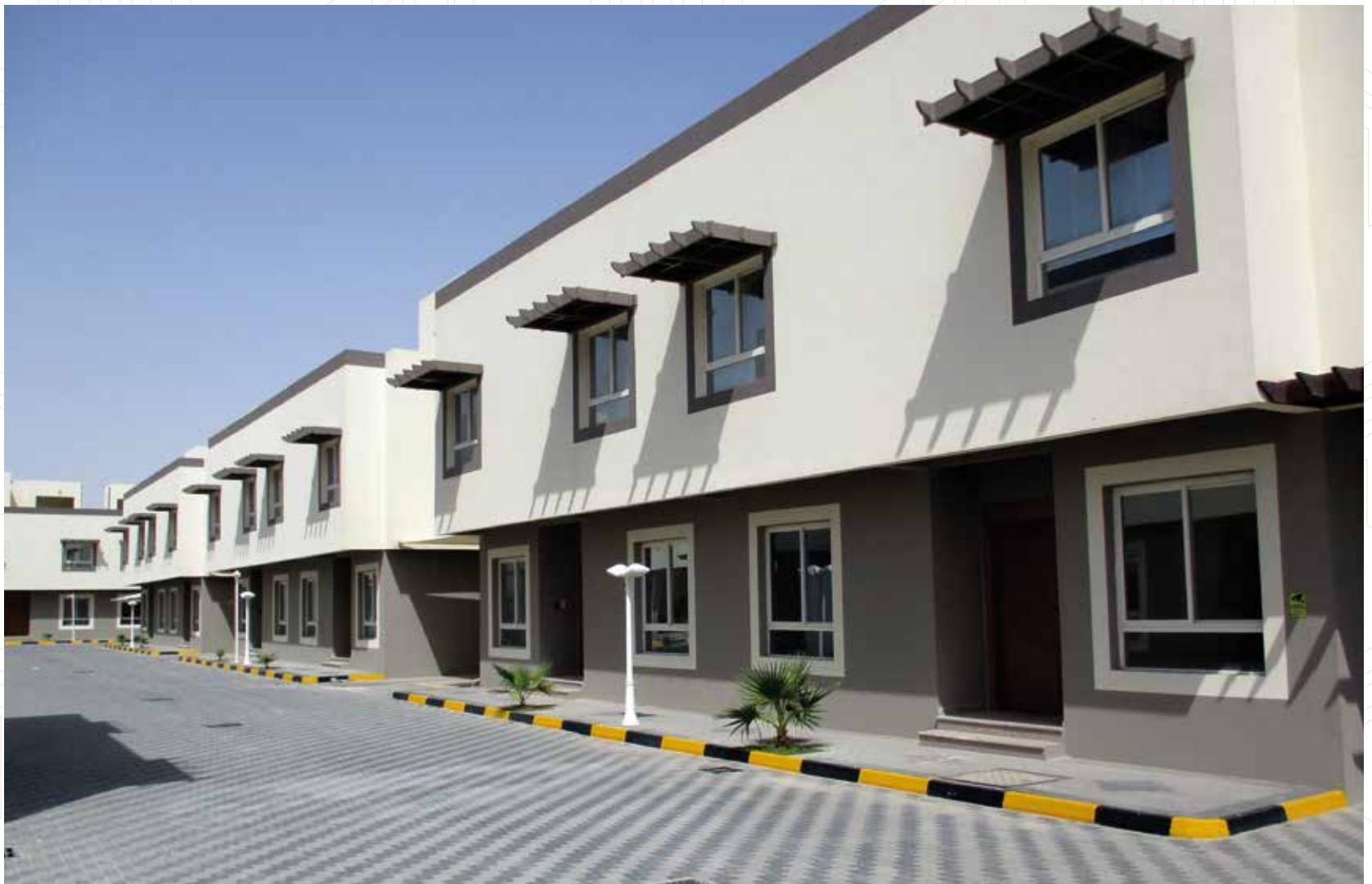
Project : 34 Villa Compound + Club house Scope : Construction and Finishing Work cities Area : AL Khisa
