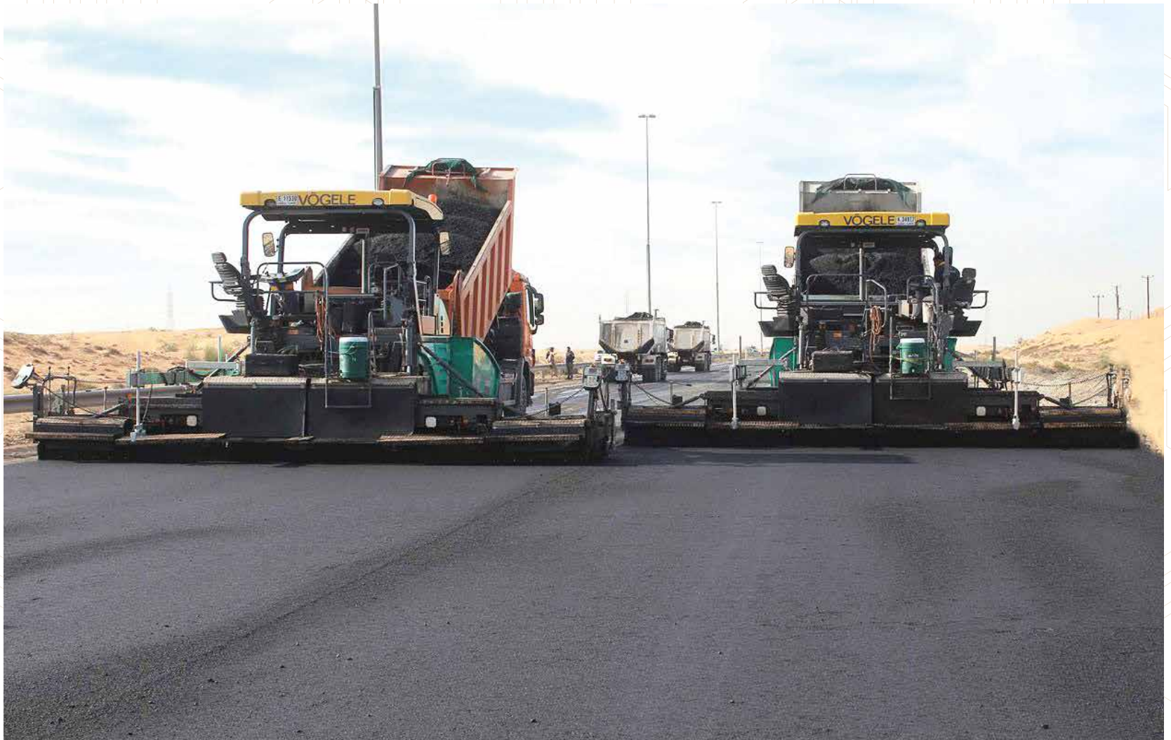
Project : Ashgal - Gleaa Street Scope : Road asphalt works Area : Doha
