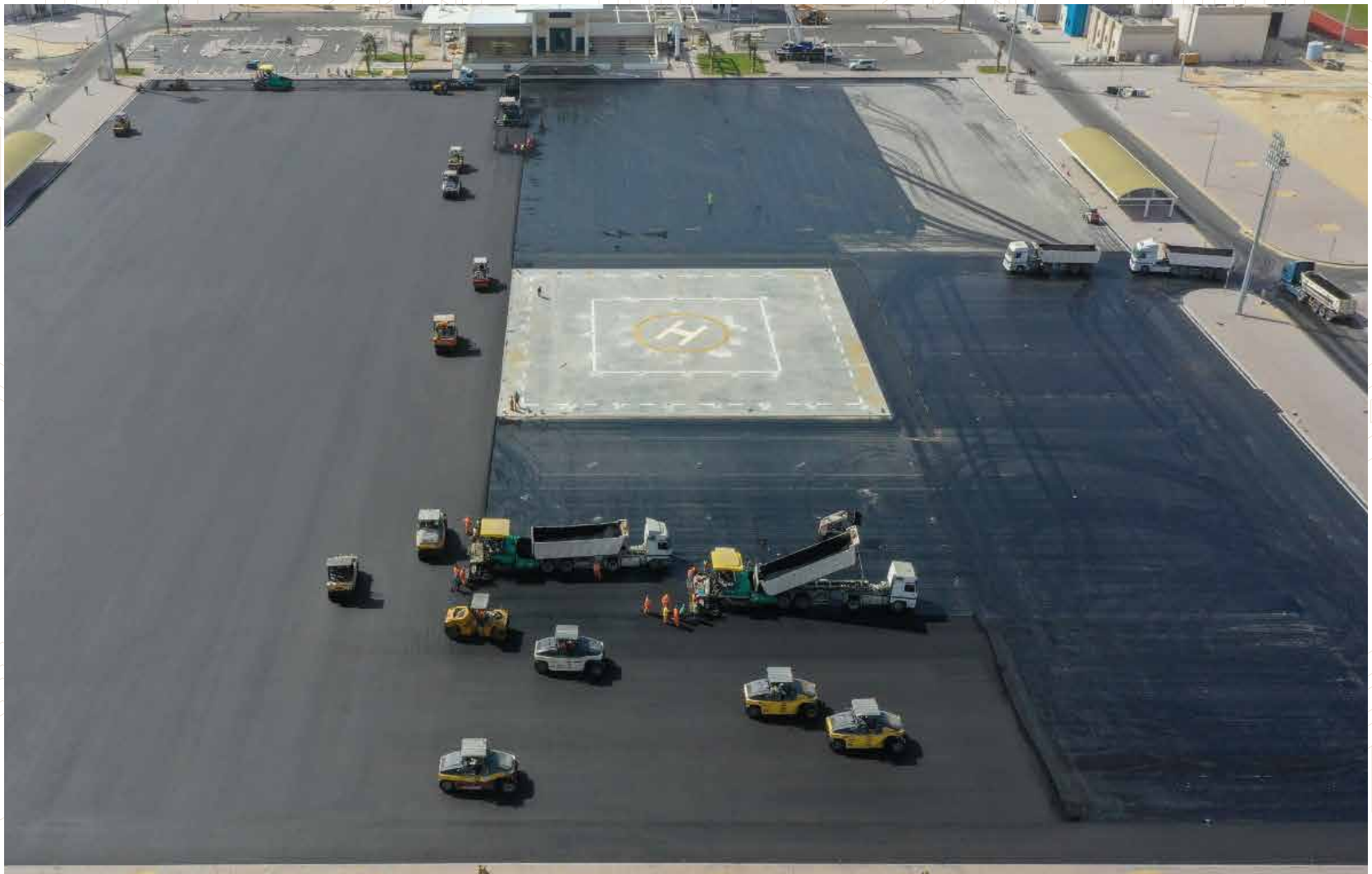
Project : Al Busair camp Scope : Road Asphalt works Area : AL Busair
