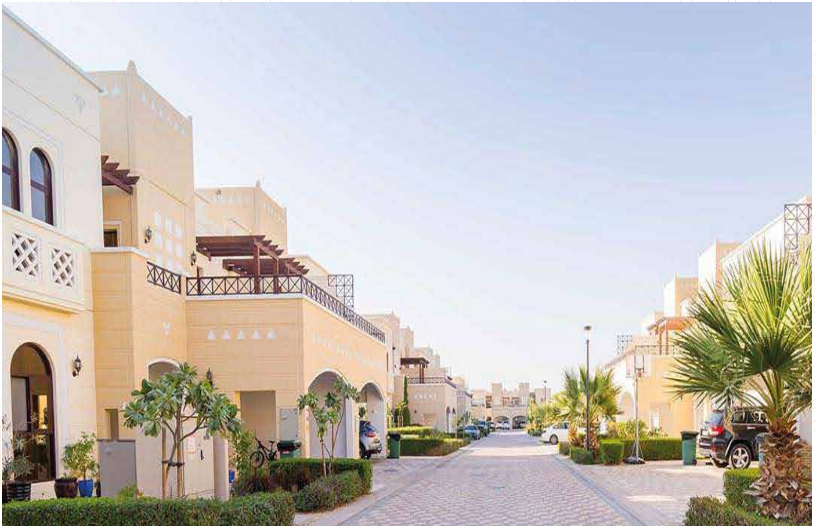
Project : Al Waab Compound Scope : Build + Finishing 56 Villa Area : Al Waab Area
