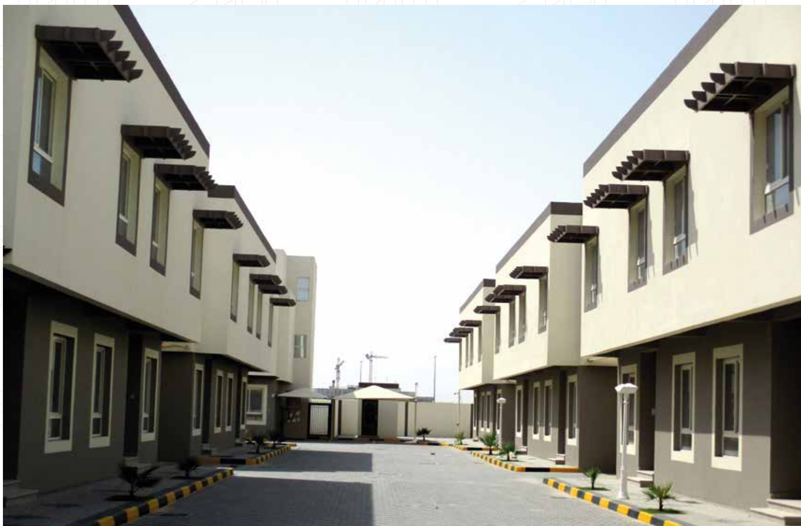
Project : 34 Villa Compound + Club house Scope : Construction and Finishing Work cities Area : AL Khisa
