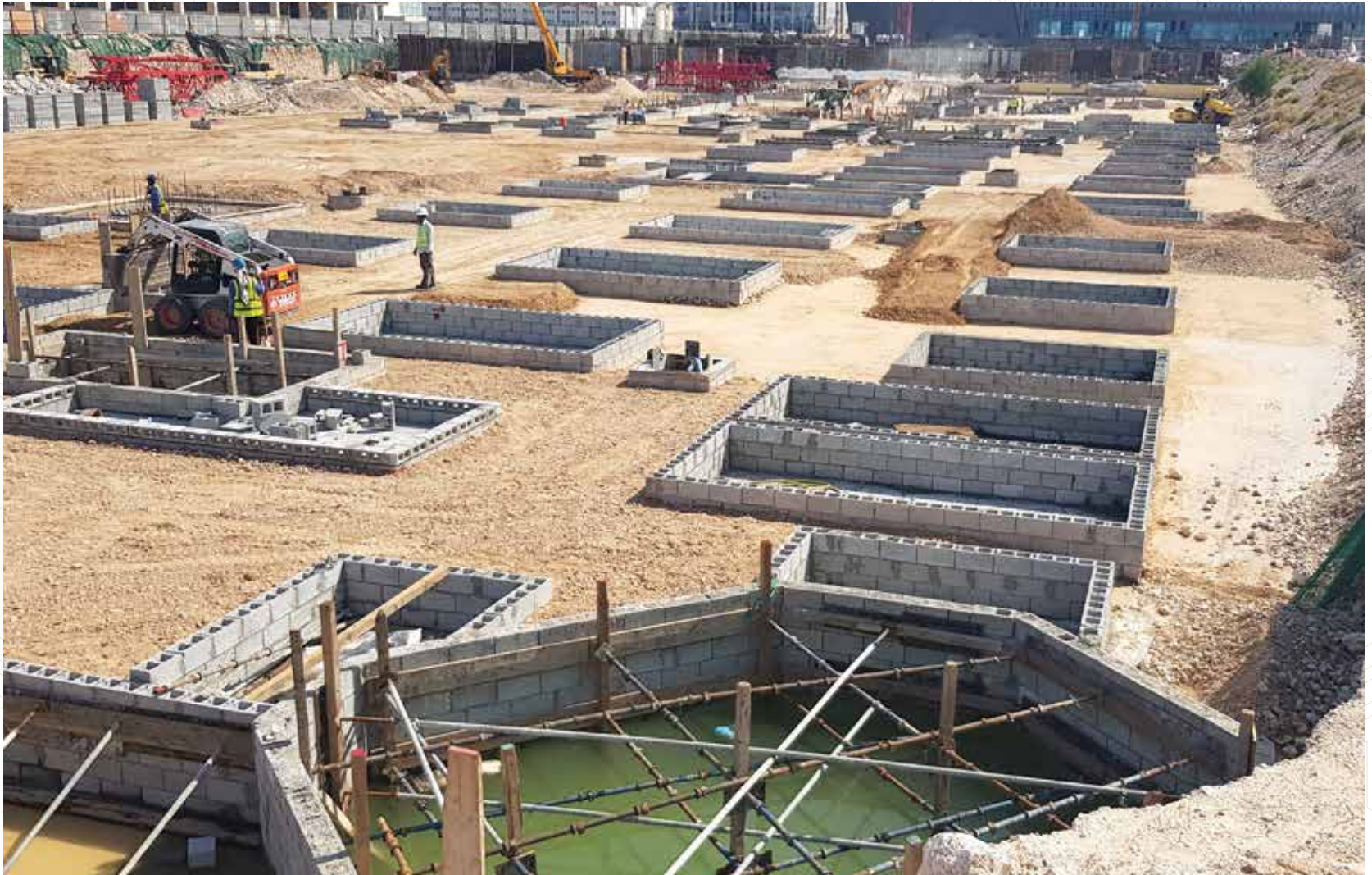
project : Al Waab Commercial Building Scope : Foundation Works (Supply & Laying of subbase) Location : Al Waab City
